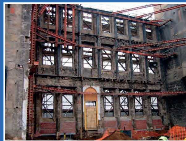
PAINSTAKING RESTORATION: The £12.5million project in 2005 was a massive undertaking.
