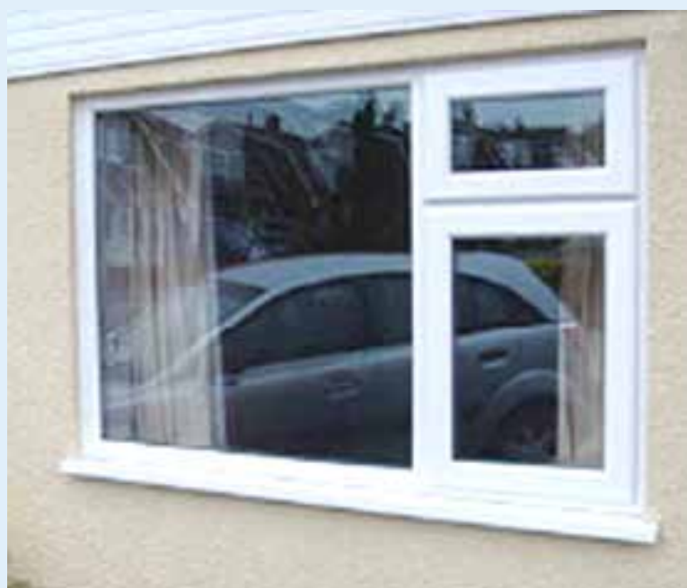
Inappropriate UPVC Window
