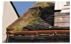
Watch out for plant growth as this can collect at parapets, skews and gutters. The plants hold the moisture and can lead to frost attack and their roots can expand and damage the stonework.
