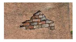
Linostone was a resinous material applied to stonework to improve appearnace in the 1970s and 80s. It does not allow the stone to 'breathe' or let moisture in the stone naturally dry out. This leads to further damage of the stone.
