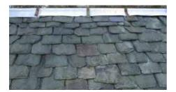
Slates are often 're-dressed' when reslating existing roofs. This causes the slates to reduce in size, which can lead to poor coverage. Ridging is essential in securing and protecting the top row of slates.
