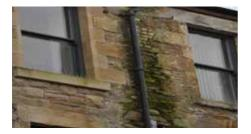
The growth of algae on stone is a sure sign that the gutter or downpipe is defective. Water concentrated on an area of stone can cause rapid decay.
