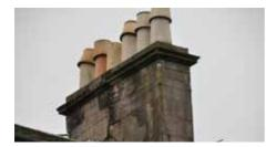
Chimneys are the most exposed parts of the building. Check that the coping is well pointed and throws water away from the face of the chimney. Render and structural defects are common on chimneyheads and falling debris can present a serious health and safety hazard.
