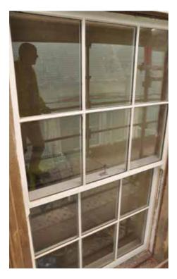
If your windows are uPVC, aluminium, or simply rotten or badly configured, then replacement timber sash and case windows and new panelled doors can be made. Modern timber sash and case windows can be made with full double glazing and draught stripping built in. These can be appropriate on the rear of buildings, however on frontages, where appearance is important, secondary glazing may be a better solution.
