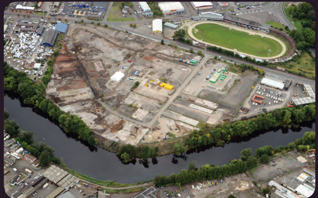
The National Business District, Shawfield
