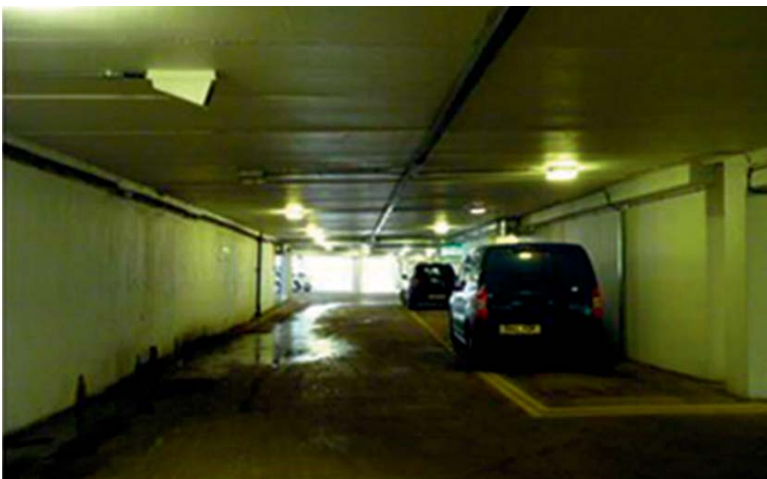
Duke Street car park before lighting project
