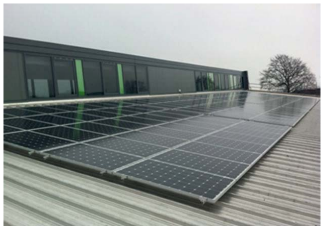
Solar panels, St Leonard's Primary School
