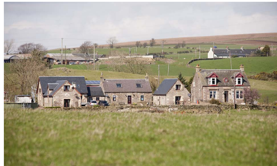
Conversion of farm outbuildings to form tourist accommodation
