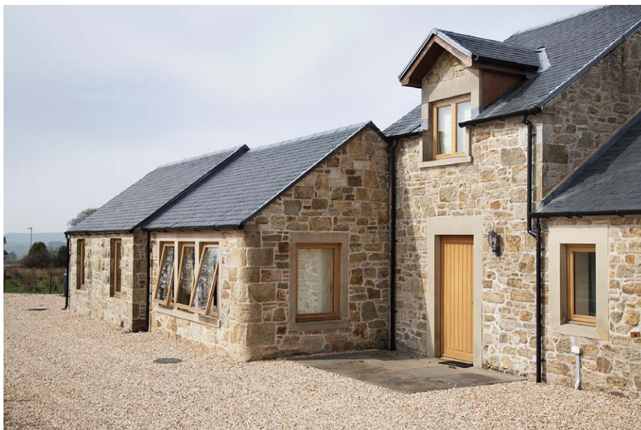
Former farm outbuildings conversion, Braehead
