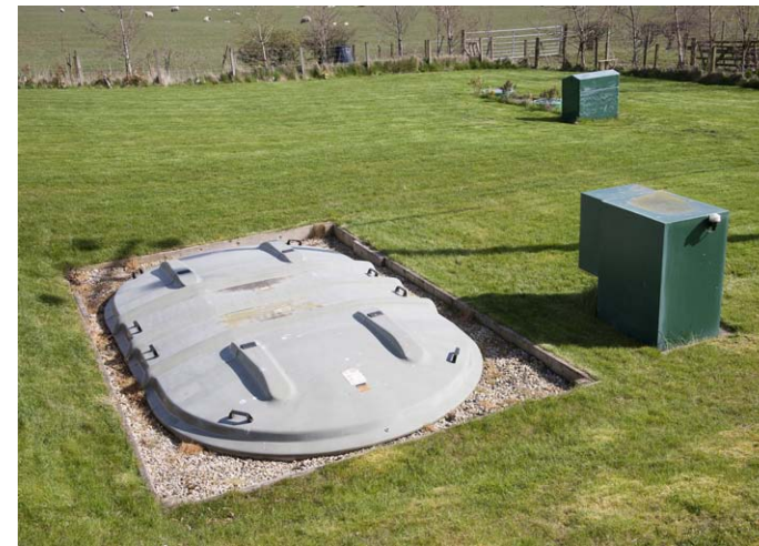
Sewage disposal by way of a biodisc system
