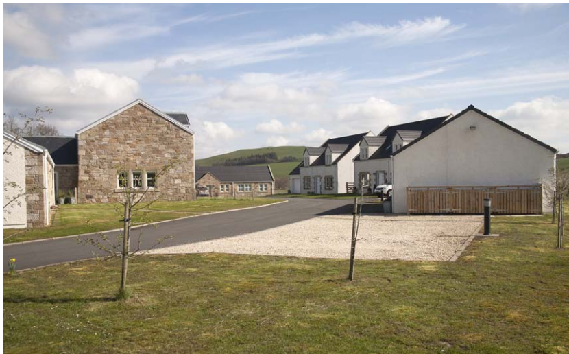
Consolidation of an existing building group
