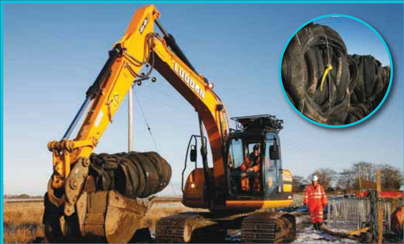
Work underway at Meadowhead Road in East Kilbride, where old tyres are being used as part of the rebuilding of the country road
