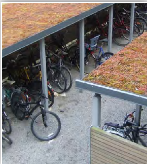
13: Bicycle storage at flatted development.
