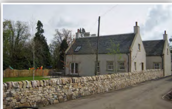
I 5: Boundary treatment creating sense of ownership.
