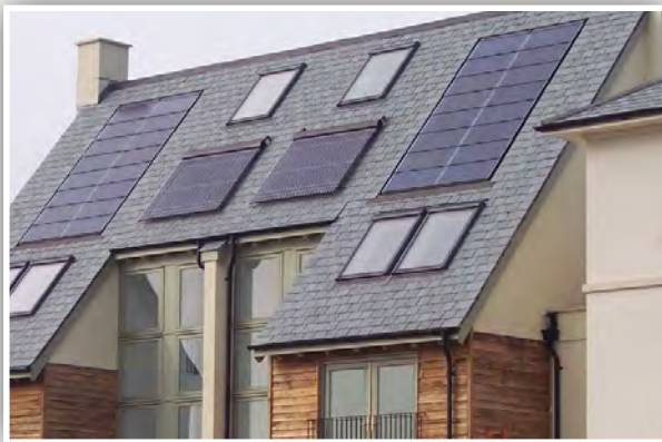
7: Incorporation of photovoltaic panels.
