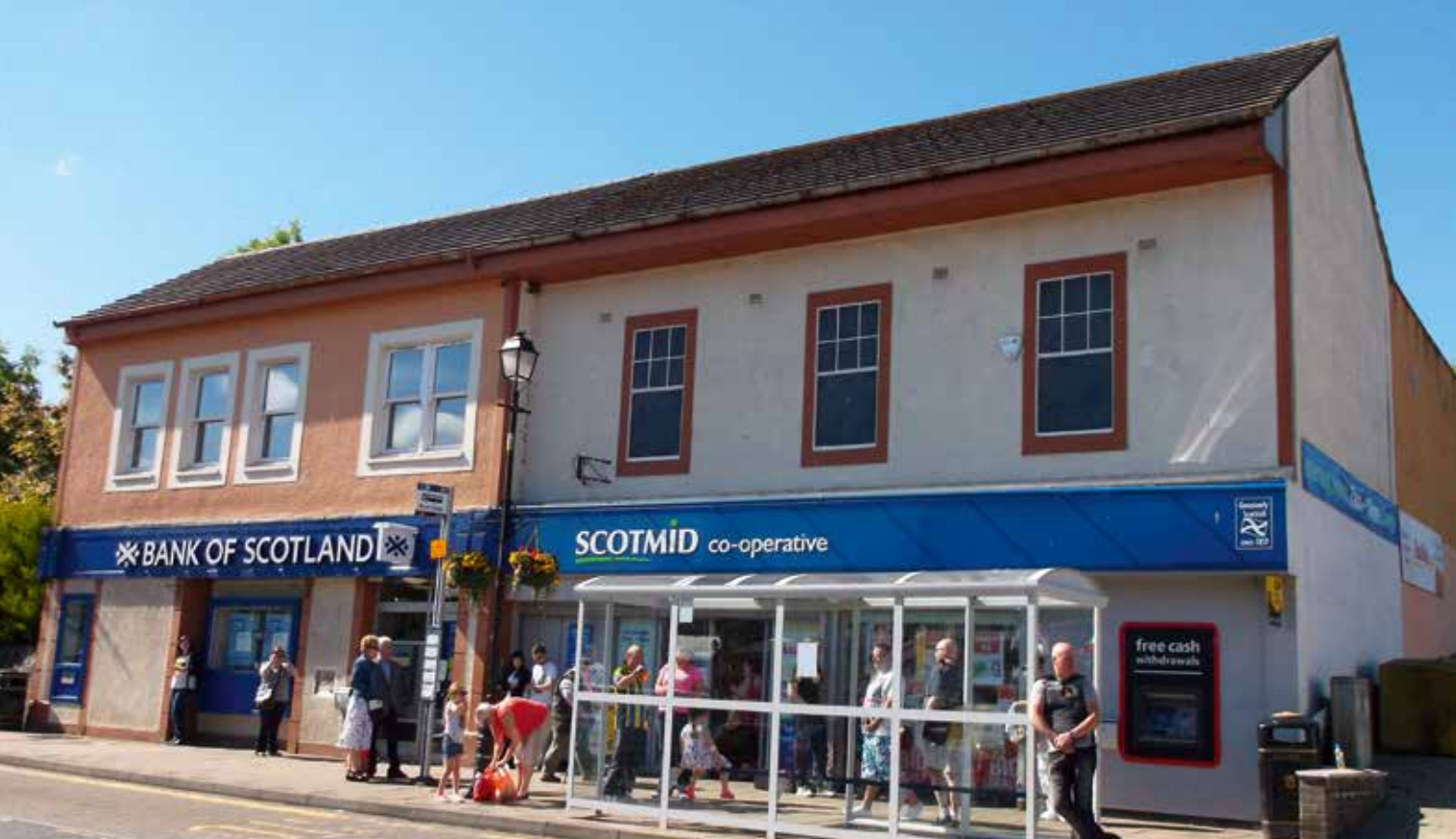
Figure 4-8: Strathaven, Common Green 1969 infill building, July 2014 (Peter Drummond Architects)
