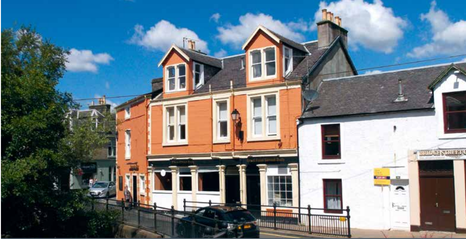
Figure 5-5: Strathaven, 6 Waterside Street, The Star Inn, July 2014 (Peter Drummond Architects)
