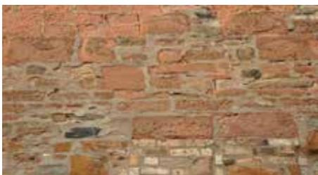
Cement pointing (here poorly done), will entrap moisture and lead to decay of the adjacent stonework. Lime pointing should be used and ideally formed to match the original lime pointing.
