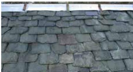
Slates are often 're-dressed' when reslating existing roofs. This causes the slates to reduce in size, which can lead to poor coverage. Ridging is essential in securing and protecting the top row of slates.
