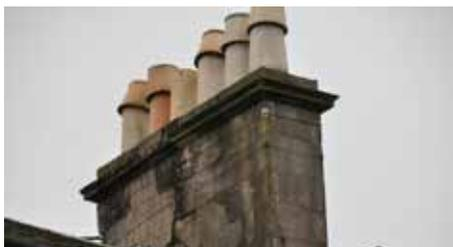
Chimneys are the most exposed parts of the building. Check that the coping is well pointed and throws water away from the face of the chimney. Render and structural defects are common on chimneyheads and falling debris can present a serious health and safety hazard.
