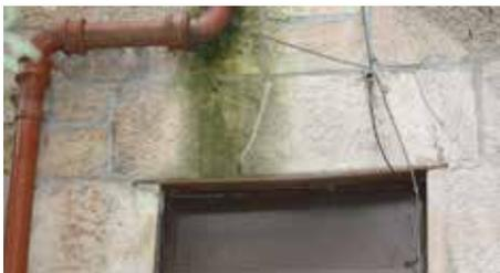
Evidence of moisture at a cracked stone lintel which has previously been repaired with a flat steel bar. Cracked lintels where moisture is evident may suggest that the timber safe lintels embedded in the wall are affected by rot.
