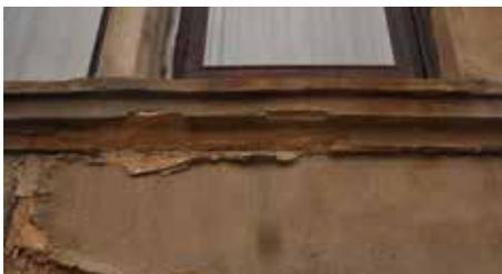
Linostone was a resinous material applied to stonework to improve appearance in the 1970s and 80s. It does not allow the stone to 'breathe' or let moisture in the stone naturally dry out. This leads to further damage of the stone.
