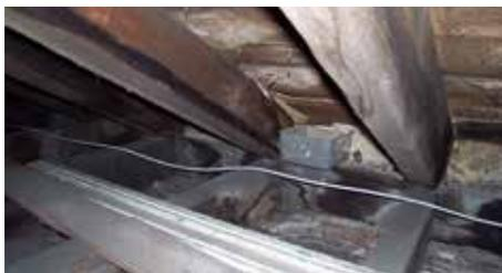
Check the loft space if it can be accessed. Water penetration behind chimneyheads and from overflowing gutters can rot the main roof timbers.
