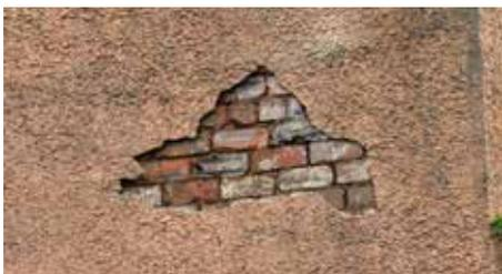
Cement based renders and roughcast can also damage the backing stone or brick. Such renders prevent the wall drying out, frost attack behind the render will fracture the render resulting in 'boss' areas and eventually cause the render to loosen.
