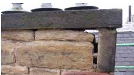
Some modern copings don't provide sufficient protection to the chimneyhead. Decayed stone and open joints can be difficult to spot from ground level.
