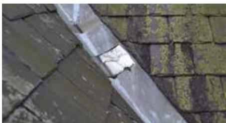
Any evidence of patch repairs to lead flashings suggests that the lead has cracked, possibly because allowance has not been made for the lead to expand and contract. Best to renew the flashings.
