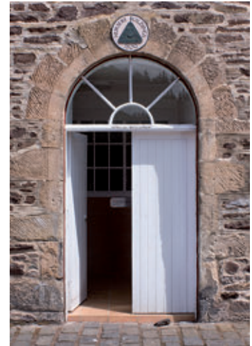
Door surround New Buildings, and fanlight detail Nursery Buildings
