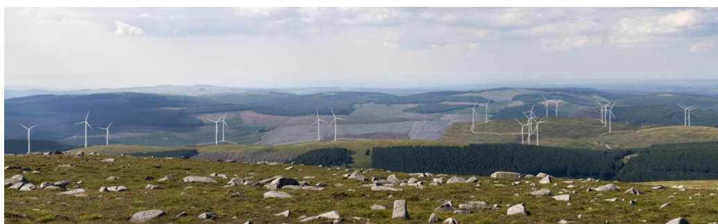
Windy Standard III Windfarm (Photomontage): the closer turbines are 125m and those further away 177.5m. Seen from Cairnmore of Carsphairn the difference in size is not apparent due to the similar proportions of the turbines and the lower ground elevation of the taller turbines
