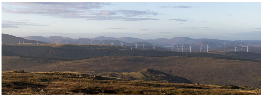
Windy Standard I and III Windfarms (Photomontage) 18 : three sizes of turbine (55m, 125m and 177.5m. Seen from Blackcraig Hill the differences in size are clear
