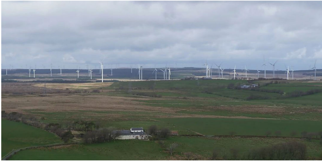
Calder Water and Whitelee Windfarms, South Lanarkshire: The more distant turbines are 110m tall. The closer turbines are 145m tall. The size difference is perceptible but not overt due to the sheer number of turbines.
