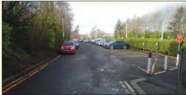
Figure 2: Station car park
