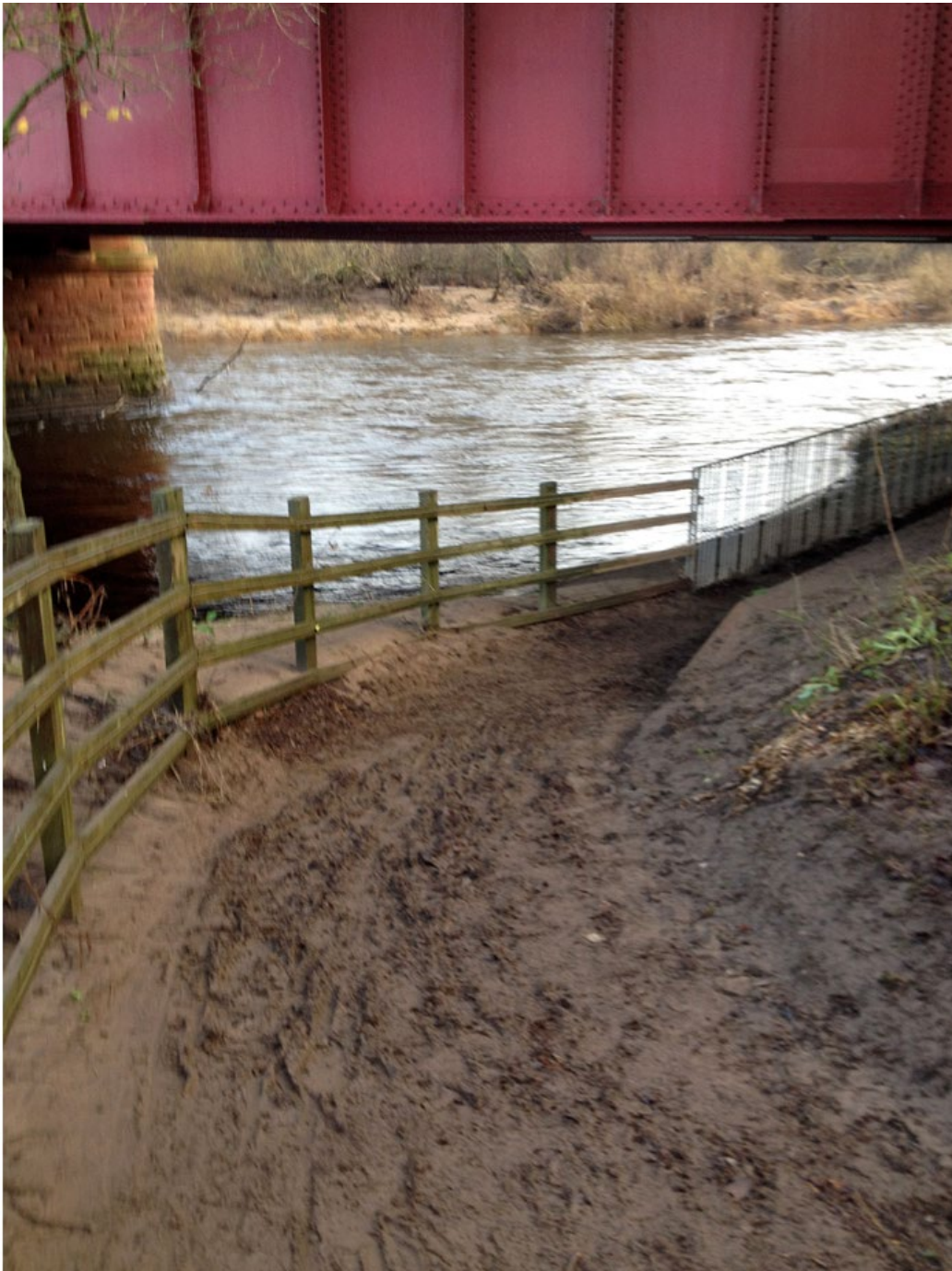
Figure 2. Muddy path under A723 bridge
